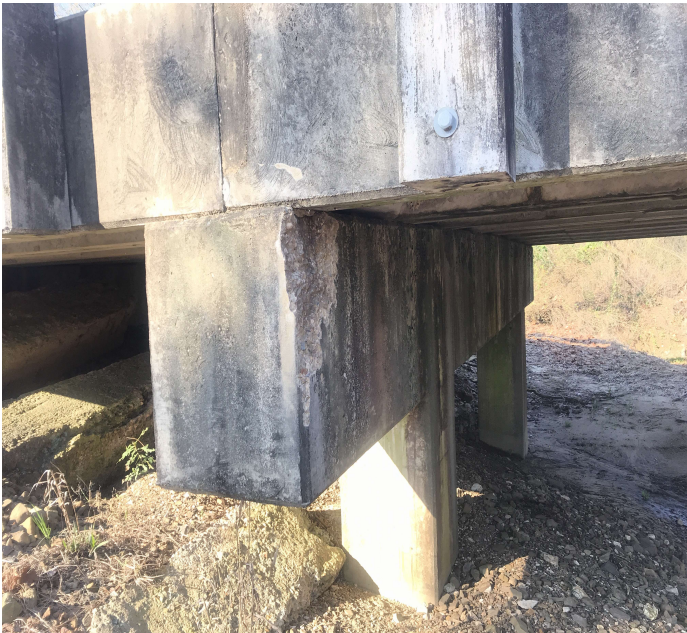
PHOTO 1 Description Spall Bent #5 left side on cap
