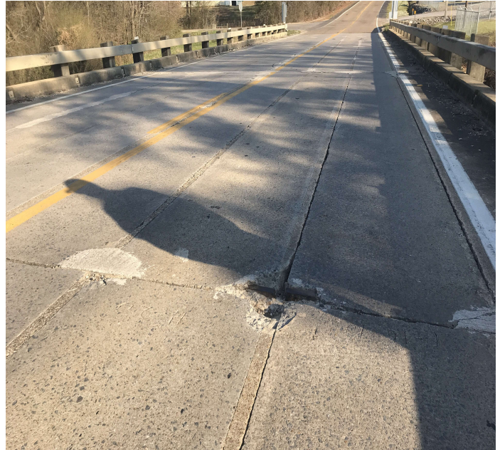
PHOTO 5 Description Spall at joint #5 corners of units are spalled at joints 2 and 3
