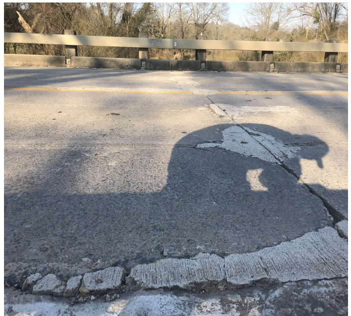
PHOTO 2 Description Joint 3 patch unsound
