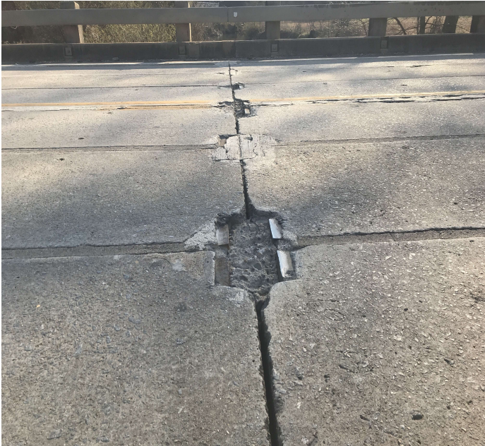
PHOTO 3 Description Joint #4 Spall joints #2,#3,#4 have spalls with metal exposed
